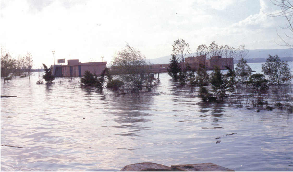
Figure 11. Inundated area due to normal faulting and lateral spreading in Kavaklı district of Gölcük town.
