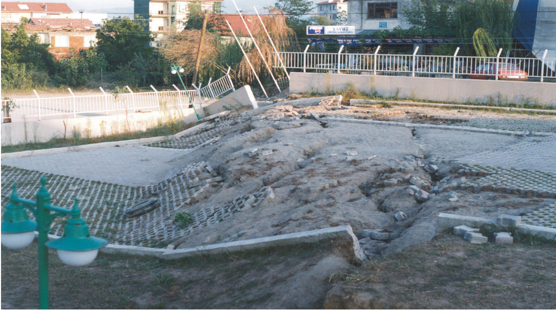
Figure 9. Flexure scarplet and left stepping en-echelon cracks along the oblique faulting in Kavaklı district of Gölcük town.
